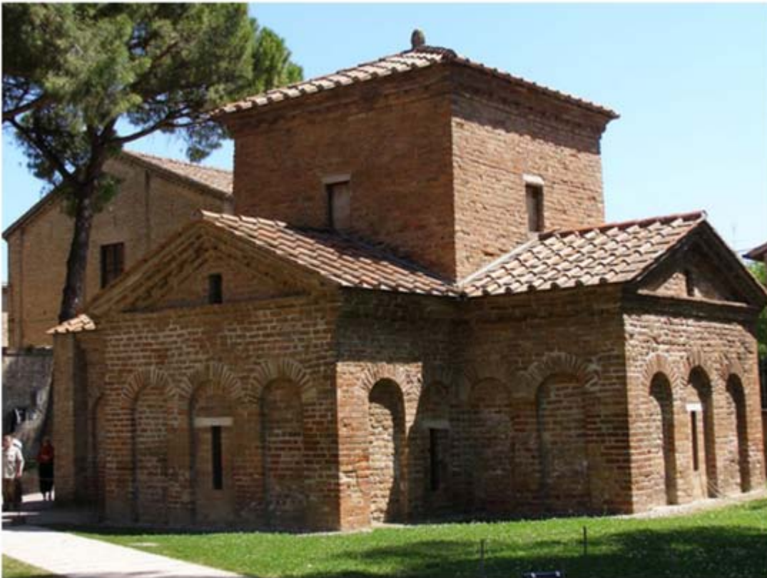
mauzoleum Gally Placidie Ravenna
